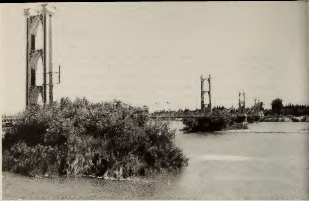
A suspension footbridge over the Euphrates River at Dayr az Zawr
